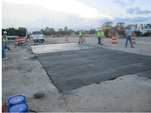
Figure 5. Finished RBMAC test pavement (foreground) and conventional PCC control pavement (background)
