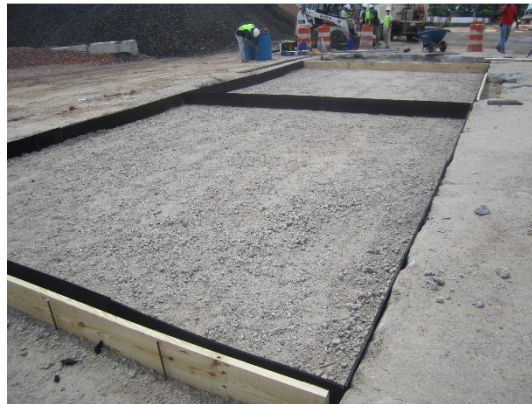
Figure 4. Compacted stone base, formwork, and isolation joint material
